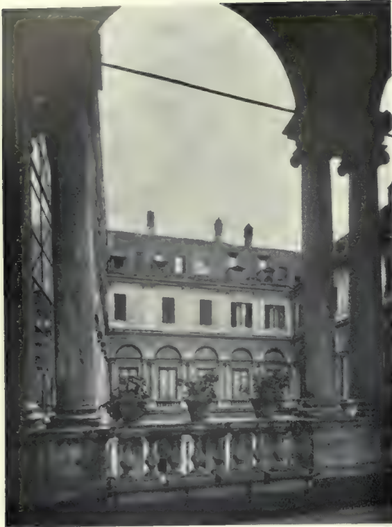
59. - Palazzo Borghese. View toward façade block from bridge loggia.
